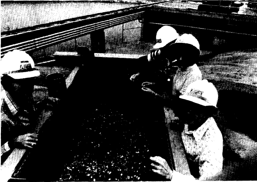
Employees of Arkansas Power & Light Co., at Unit 2 of the Arkansas Nuclear One station, near Russellville, are shown with thousands of Asiatic clams being removed from the intake bay of the plant's cooling water system. The unit had to be shut down because of inadequate flow of service water through the containment air coolers. The freshwater clams, attracted by the slightly warmer water, had gotten into the system, grown and caused the blockage. First discovered in the United States on the West Coast in 1938, the clams have spread rapidly into at least 33 States, and have been found at virtually all of the Tennessee Valley Authority's generating stations.
