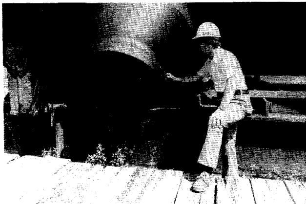
Inspections during construction of Duke Power Co.'s two units at its Catawba Nuclear Station site in South Carolina. Shown clockwise, from top left, are inspections of a pipe weld reinforcement, pipe fittings, reactor pressure vessel head con-
